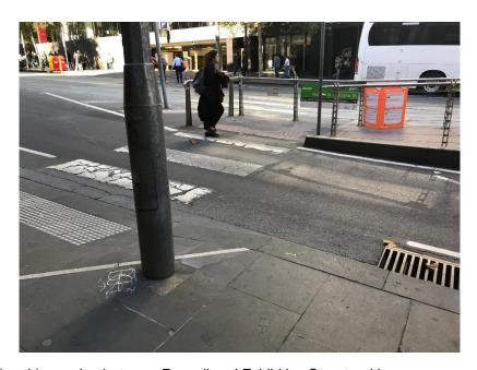
Bourke St (north) crossing between Russell and Exhibition Streets with pram ramp extending into footpath reduces footpath width and creates potential trip hazard.
